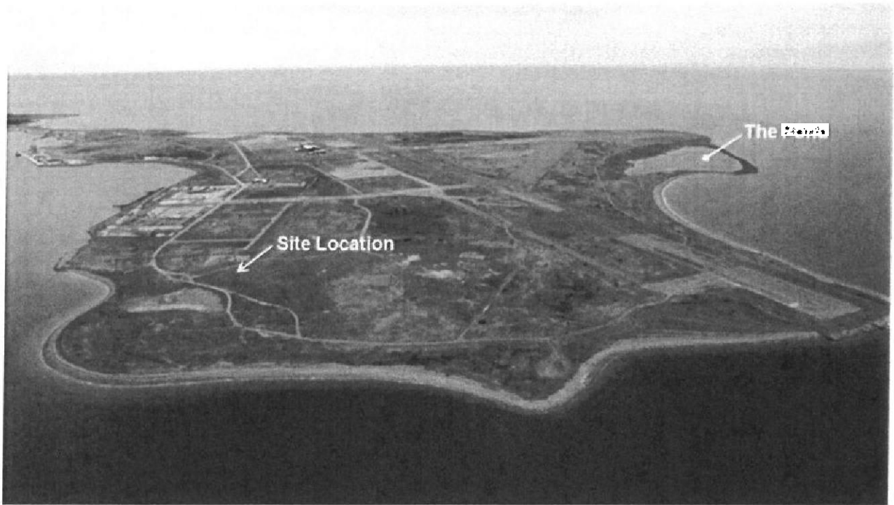
Figure 1.1b: Construction Site looking south-west
